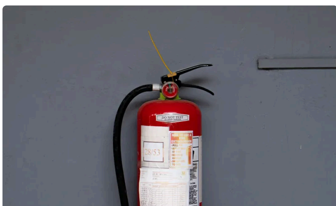
P2. CO2 extinguisher on the floor outside the café. Ground floor corridor, 09:53.
